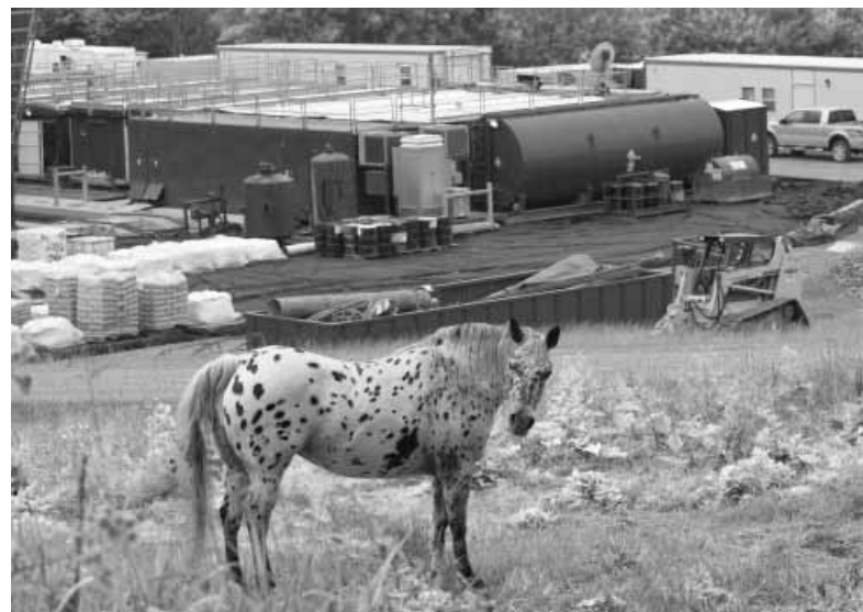
Infrastructure at the Kerr well in Lathrop Township, Susquehanna County (PA). Photo by Frank Finan
